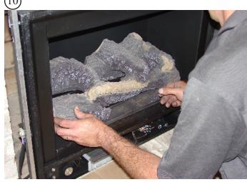
Place log set in firebox. Center the logs right to left and push back against the log stop.
