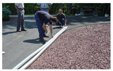
Uncoil the three inch aluminum chimney liners on the ground and measure to make sure the pipes are long enough. Mark one of the liners at both ends with paint and use it for the exhaust side connection. Once they are in the chimney it allows easier identification of intake and exhaust connections.
