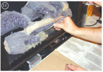
Place rock wool on burner as shown above. The wool should be placed loosely and lightly. This wool forms the glowing ember bed and will look different depending on placement. Reinstall the glass door assembly and close the latches.
