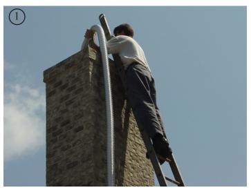
Feed chimney liners down the chimney and through the damper. If the fireplace opening does not allow enough room to connect the flue liners to the stove it is necessary to separate the exhaust/ intake pipe adapter from the stove body.
